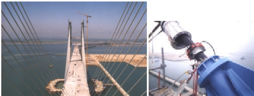
Fig. 8 Cable of Seohae Bridge and Installation of Cable Damper(DGD)
