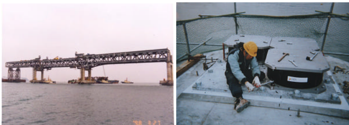
Fig. 2 Kwangan Bridge with Lead Rubber Bearing
