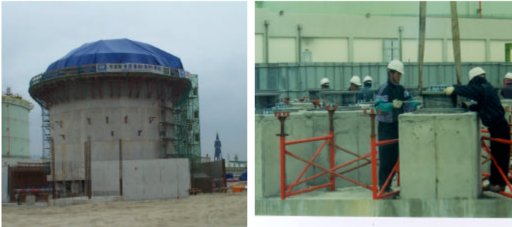
Fig. 3 Base-isolated Pilot LNG Tank under construction
